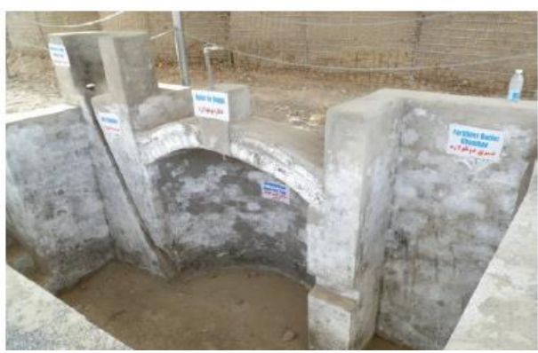
Construction of a 4 cubic meter biodigester
