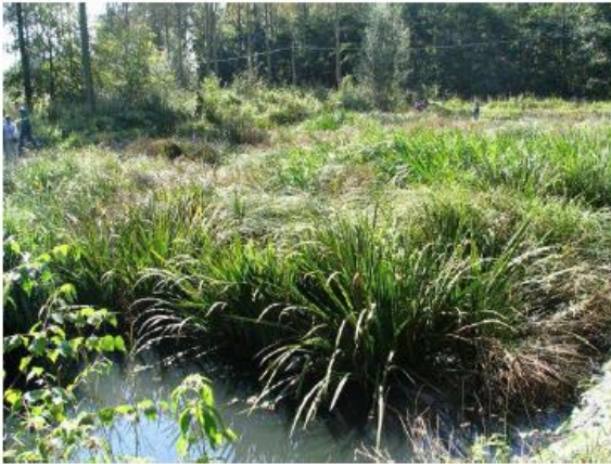
Floating wetland rafts treating for combined sewer overflows at Bornem in Belgium (Photo C.C. Tanner October 2005).
