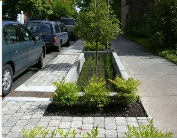
Pre-cast concrete box with a small tree or shrub planted installed along the edge of parking lot, roadway. Its primary treatment mechanisms: sedimentation, filtration, adsorption, biodegradation.
