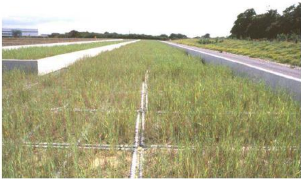
Full-scale floating treatment wetland system for removal of glycol from de-icing water at Heathrow Airport, UK.
