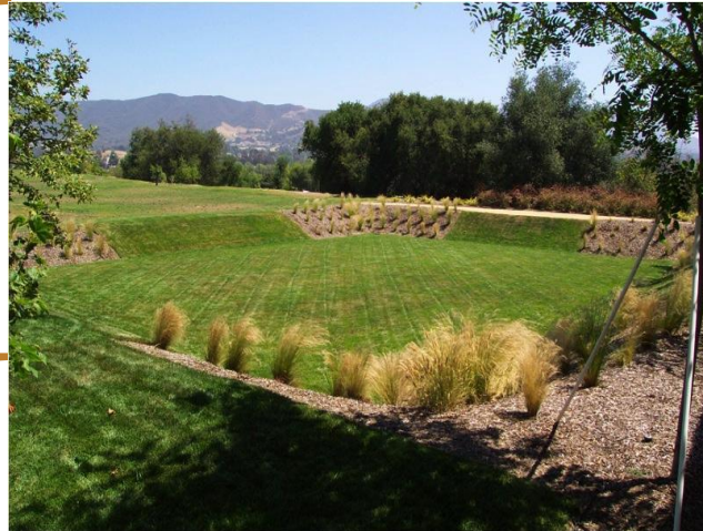
Single-stage Shallow earthen basin which is designed to retain and infiltrate stormwater runoff and its primary treatment mechanisms are filtration, adsorption, biodegradation.
